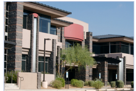
Vegetation too close to windows.
